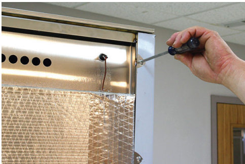
Figure 1: Remove top screw
