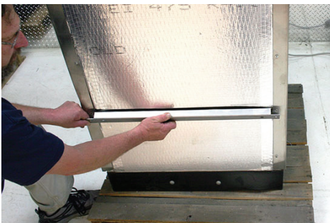
Figure 9: Install bottom seismic bracket
