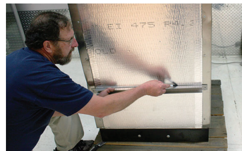
Figure 6: Align bottom bracket with holes
