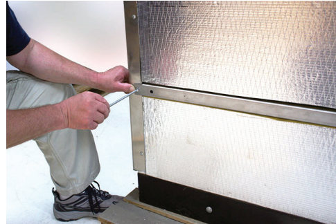
Figure 10: Re-install bottom screws – both sides
